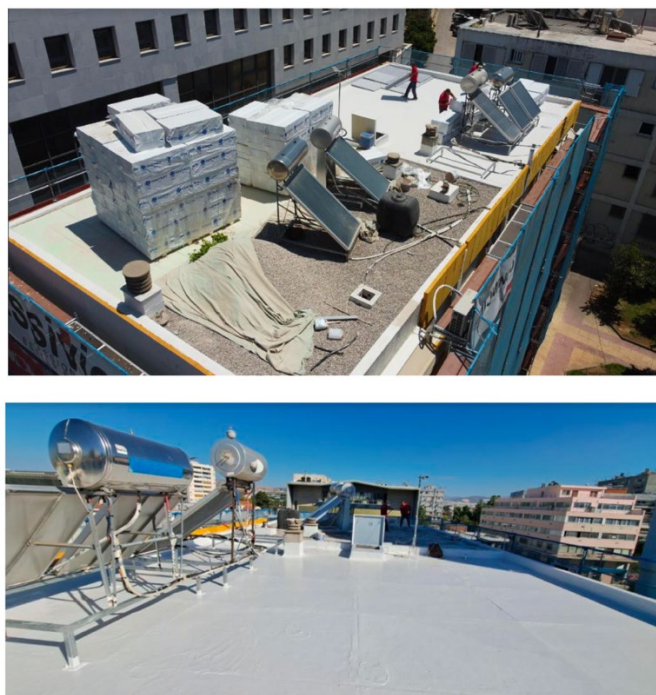
Figure 12 The roof at the Tavros project during implementation of the insulation.
