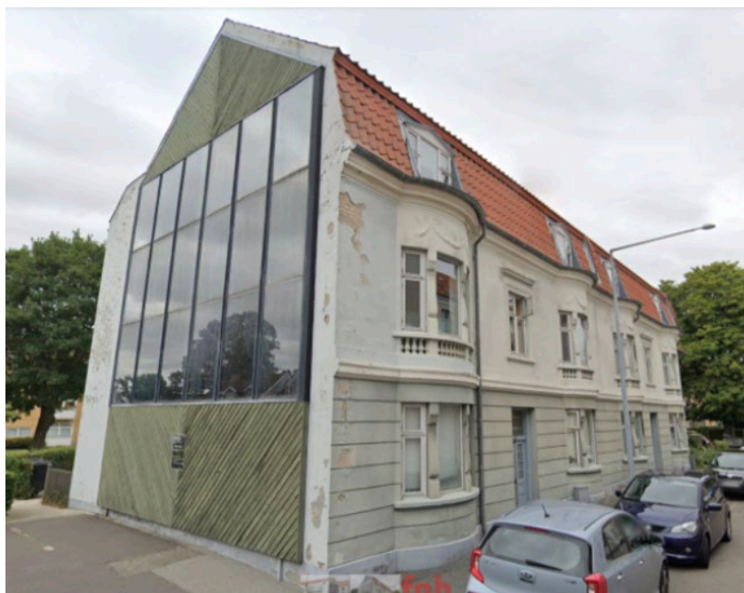
Figure 24 The gable to the South
