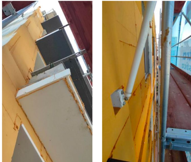
Figure 10 Insulation at the facades with RINNO technology (K-FLEX).
