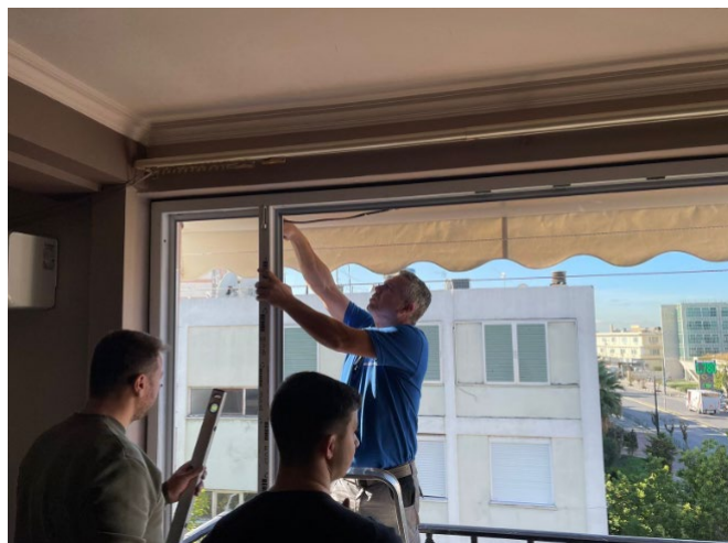
Figure 11 Installation of the Thermo-chromic glass (GREEN-STRUCT).
