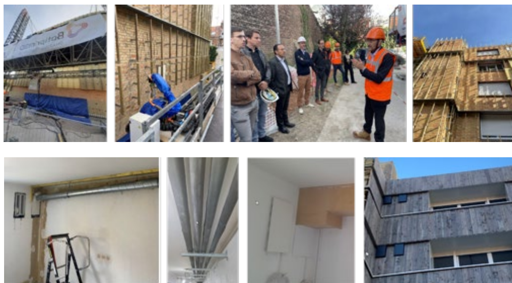
Figure 4 The RINNO works (thermal insulation and technologies implementation)
