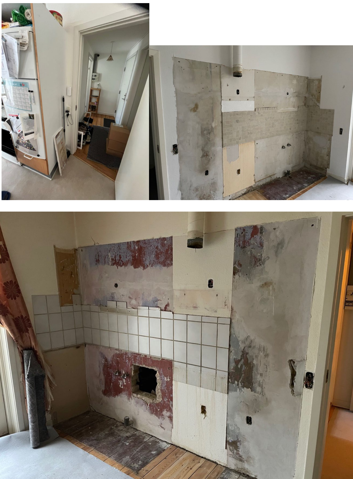
Figure 26 Ongoing renovation works at Olufsgade - January 2024
