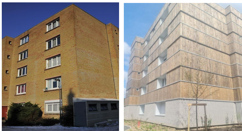
Figure 3 Photo before and after renovation
