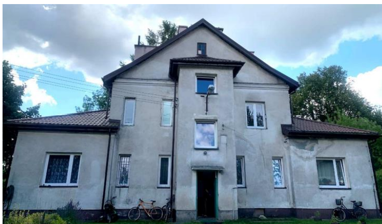
Figure 16 Poland demo building: Masovia Voivodship in Rajszew
