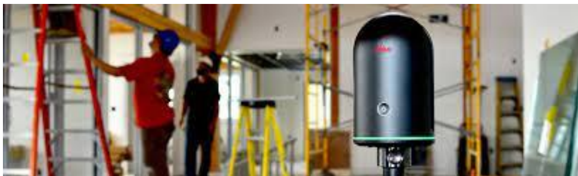
Figure 4 - Building interior using Standard LIDAR
