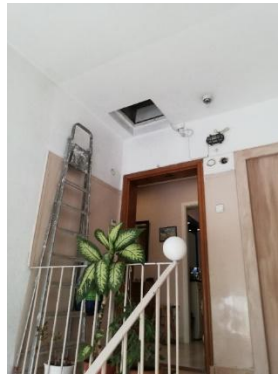
Figure 12 Access to the roof for pilot
