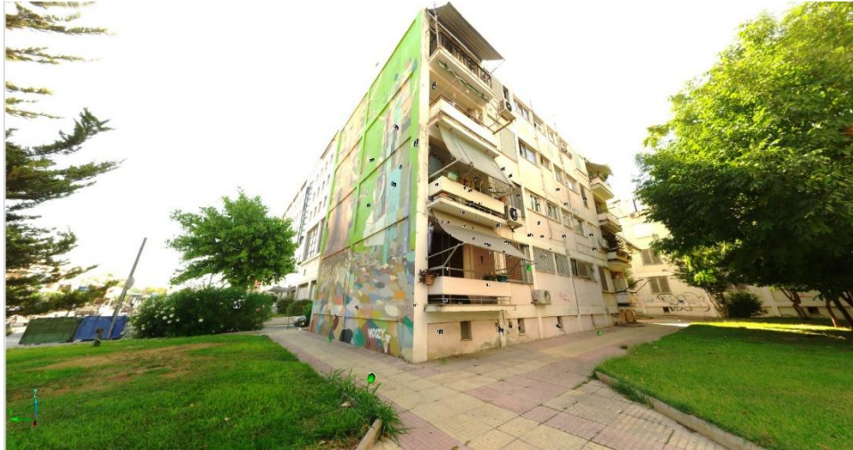
Figure 9 Greek Demo Building in Athens
