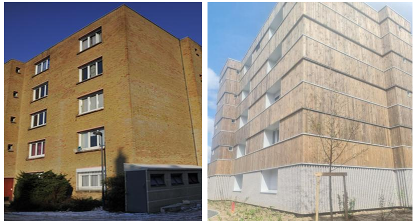
Figure 1. French case study: before (left) and after (right) renovation.
