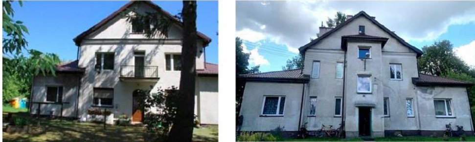
Figure 2-2: Polish demo building
