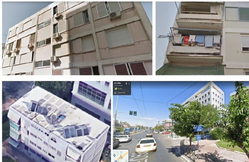
Figure 2-1: Greek demo building
