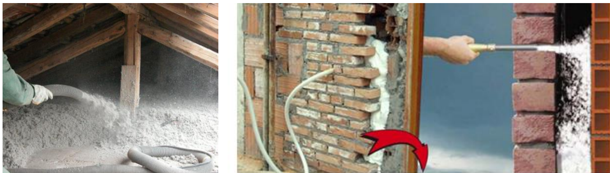
Figure 7 - ISOCELL Cellulose Insulation (CBI Danmark) and insufflation
