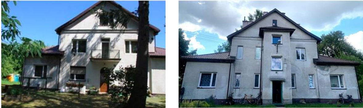
Figure 17 - Polish demo. South (left) and North (right) façades
